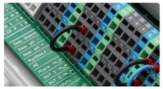
Wire bridge in the terminal box from phase LF to centre relay contact a
